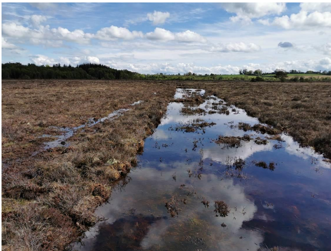
Figure 2.3 Example of contour bund constructed at Knockacoller Bog SAC, Co. Laois
