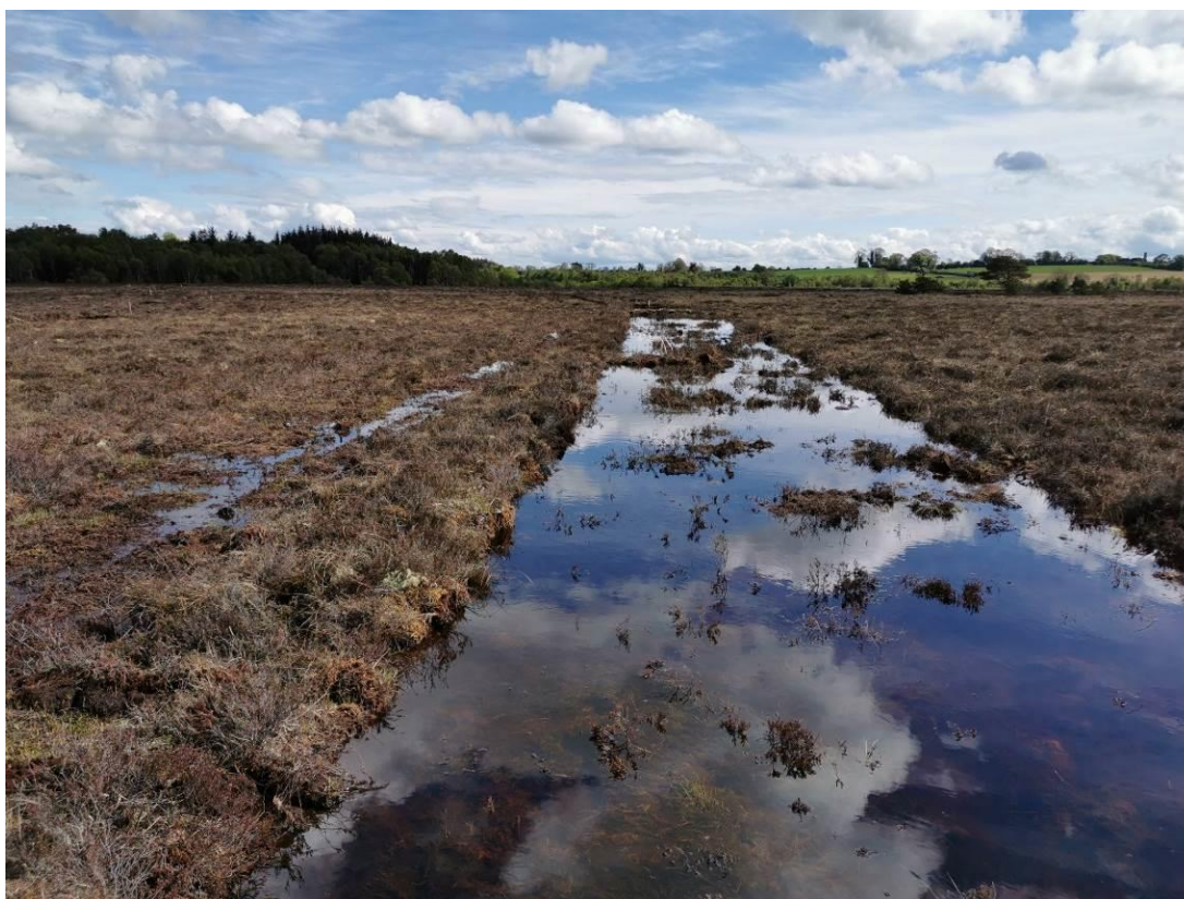
Figure 2.4 Example of contour bund constructed at Knockacoller Bog SAC, Co. Laois
