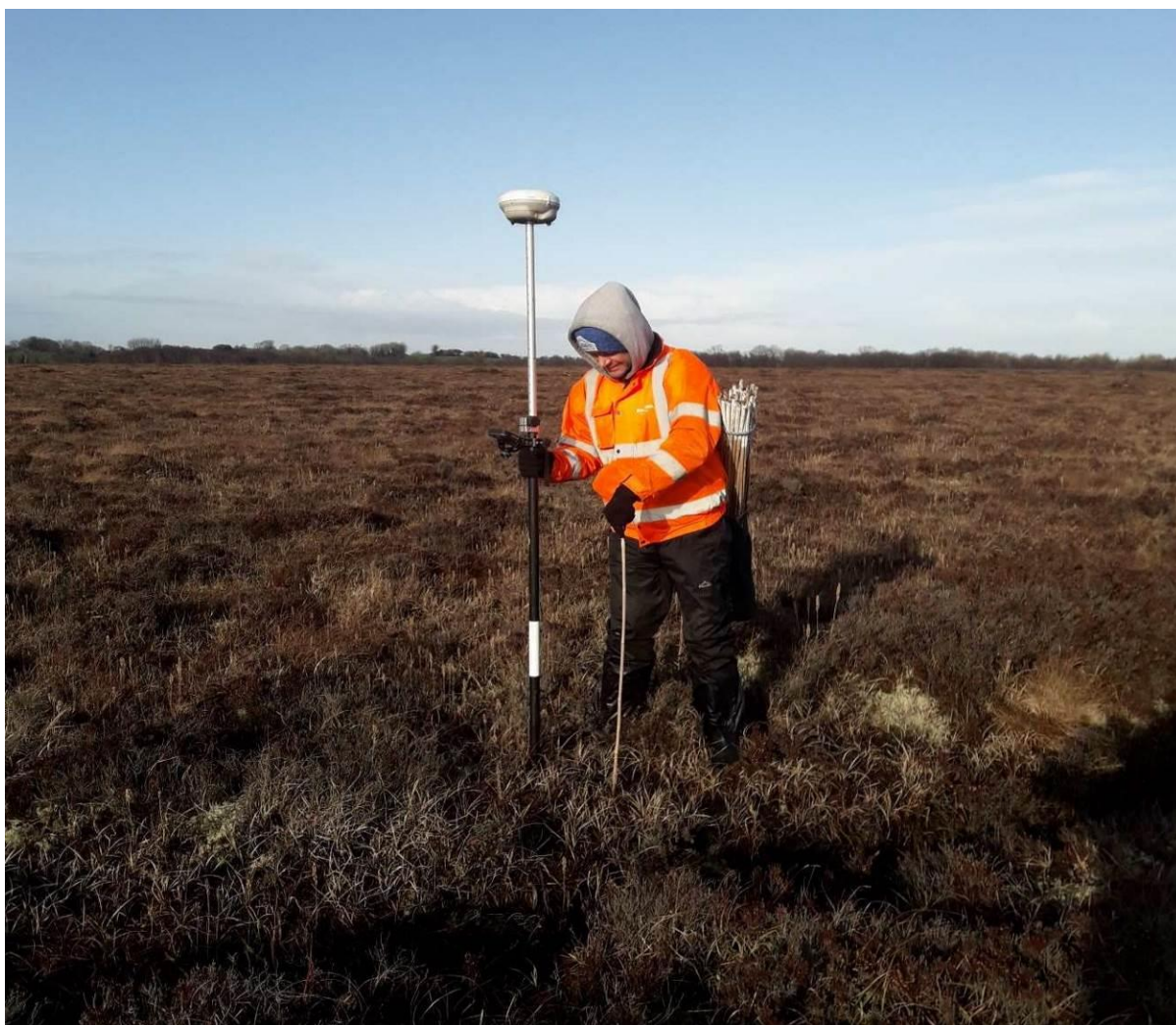
Figure 5.2 Example of setting out dams on an area of high bog
