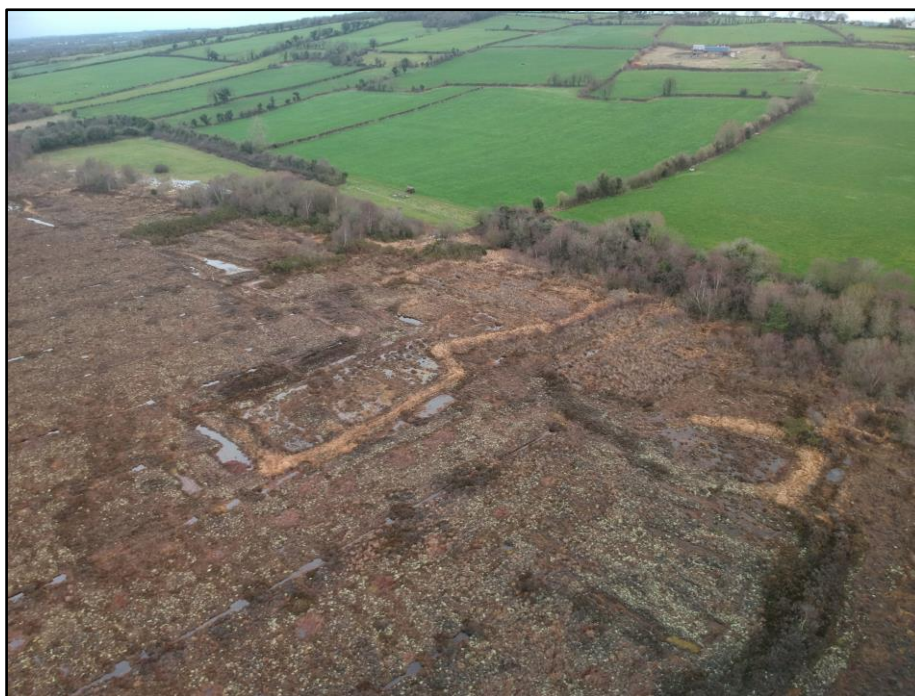
Figure 5.7 Example of drain blocking carried out on the high bog and cutover illustrating the contrast with the adjacent grassland on mineral soils
