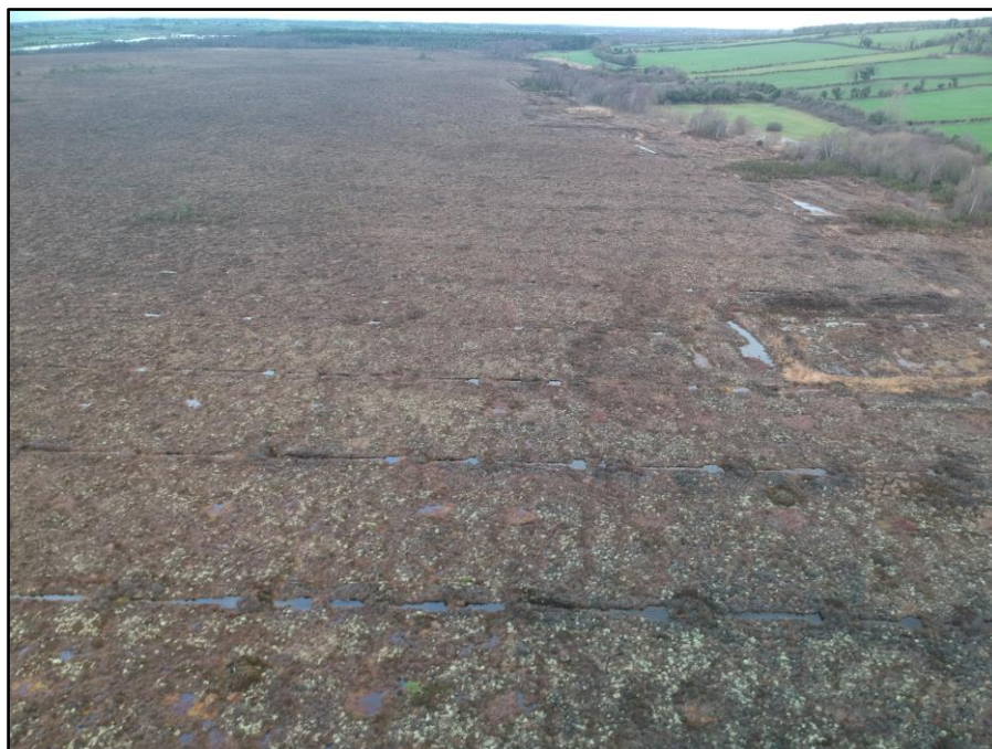
Figure 5.6 Example of drain blocking carried out on the high bog and cutover
