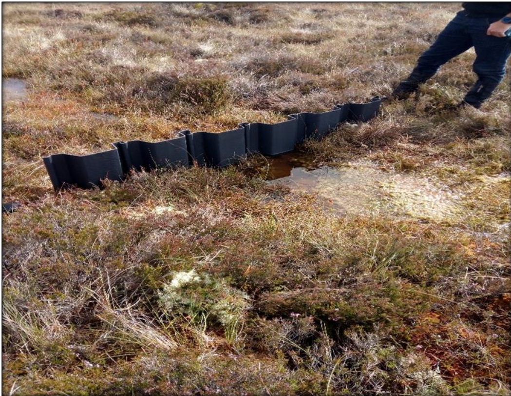
Figure 5.5 Example of plastic sheet piling installed in a drain where the machine could not reach due to wet ground conditions
