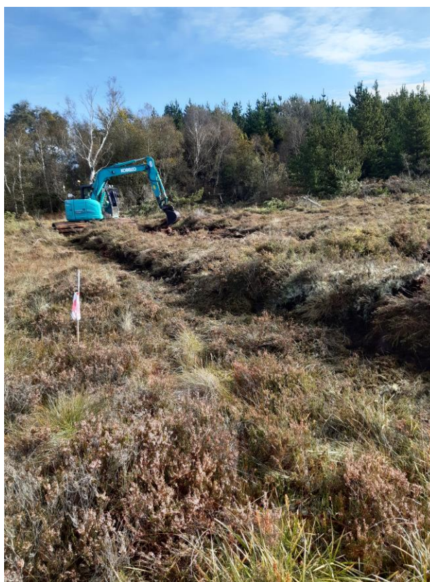
Figure 5.5 Example of setting out trench bunding on a cutover with bamboos and tape
