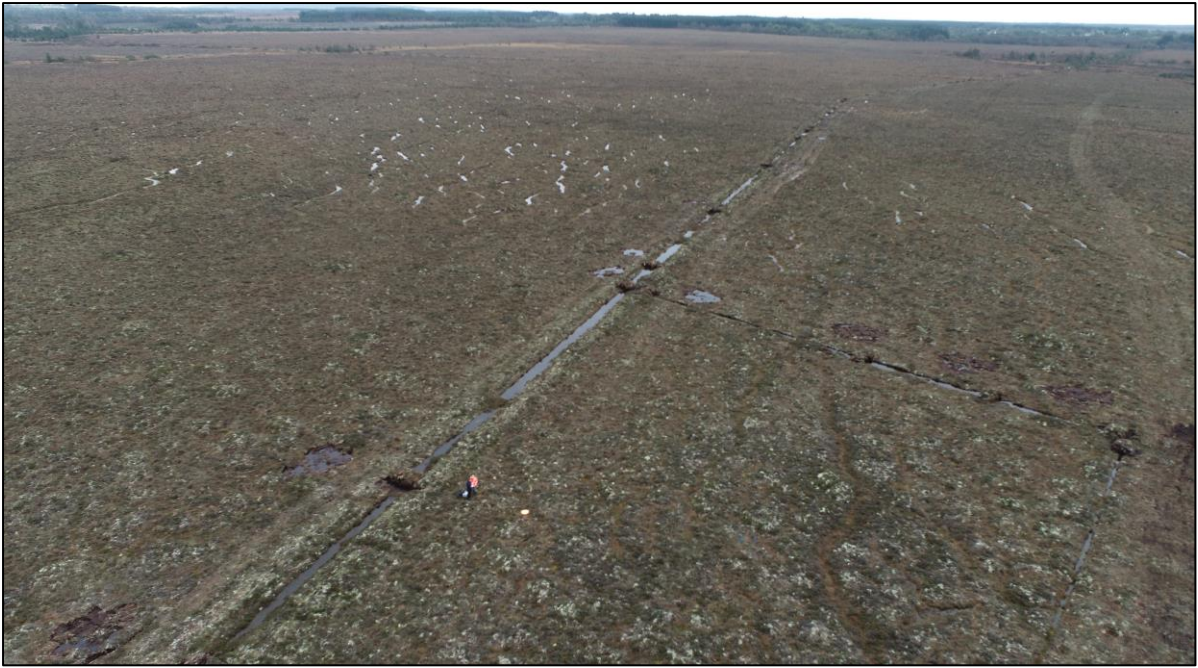
Figure 5.5 Example of drain blocking with peat dams on the high bog
