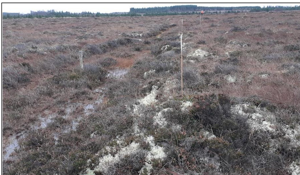
Figure 5.3 Example of setting out dams on an area of high bog
