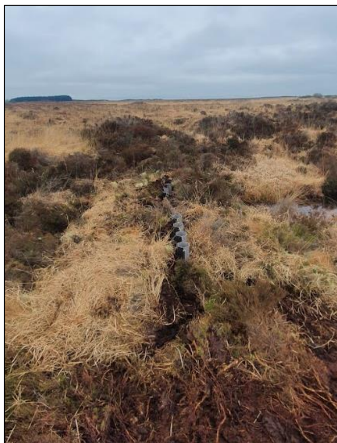
Figure 5.5 Example of plastic and peat sandwich dam constructed at Kilsallagh Bog.
