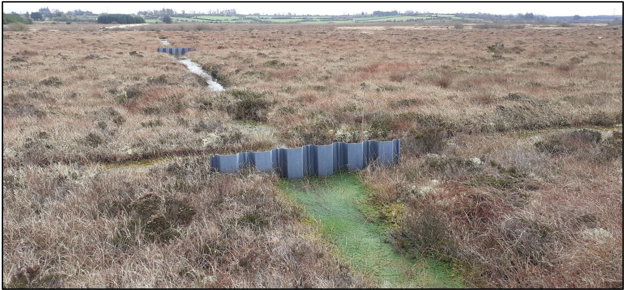
Figure 5.6 Example of plastic dams constructed at Kilsallagh Bog.
