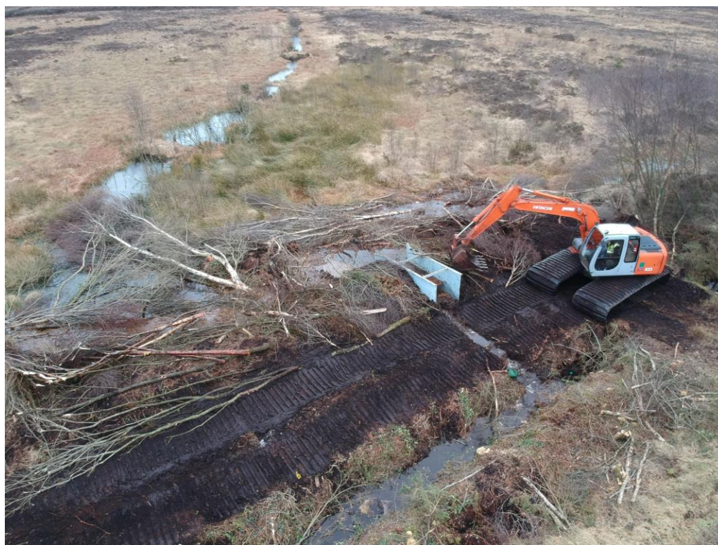
Figure 2.5 New outlet being installed in a large marginal at Killyconny Bog.
