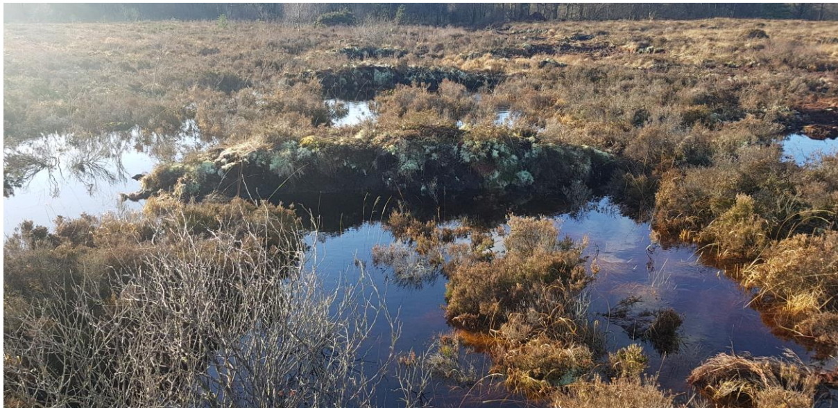
Figure 5.6 Example of peat dam installed on the cutover of Garriskil Bog
