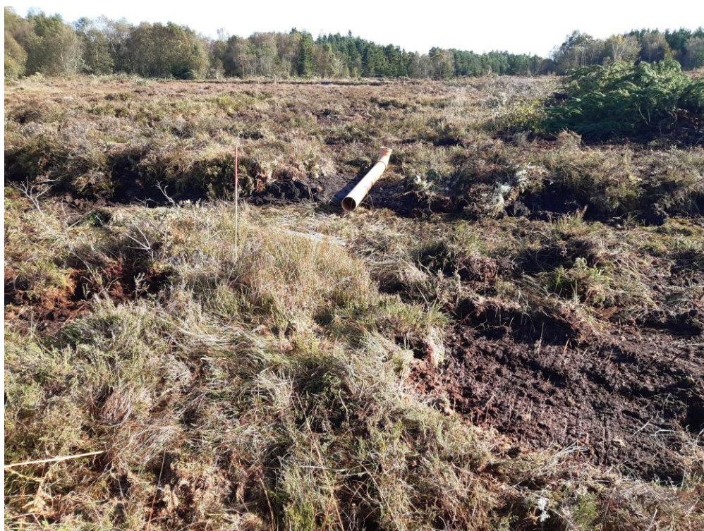
Figure 5.5 Example of setting out for piped weirs in a trench bund on the cutover. The bamboo is sprayed red
