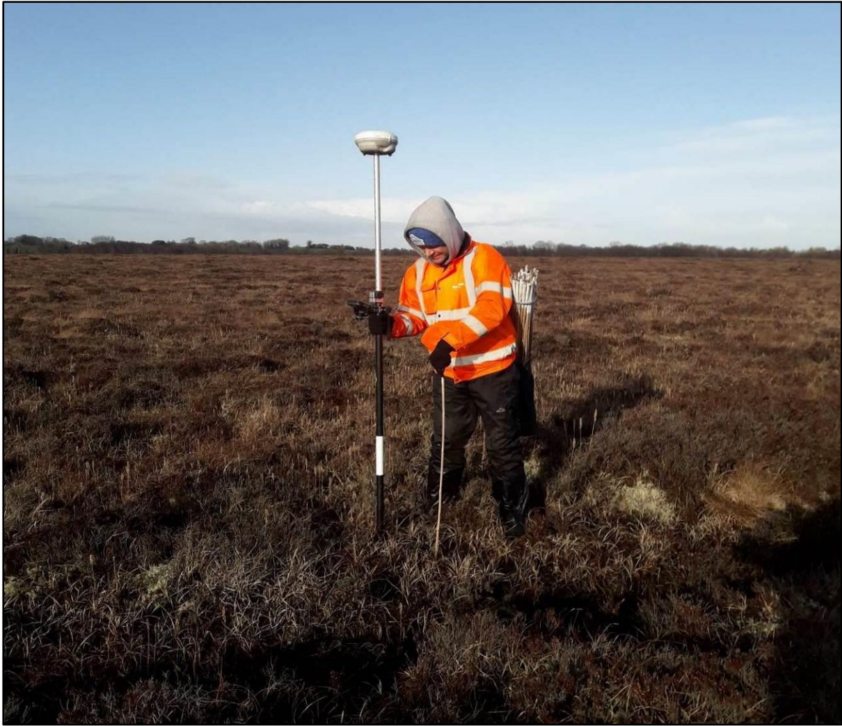
Figure 5.1 Example of setting out dams on an area of high bog
