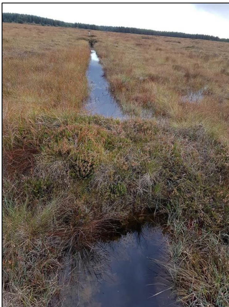
Figure 2.1 Example of a peat dam used to block a typical high bog drain.
