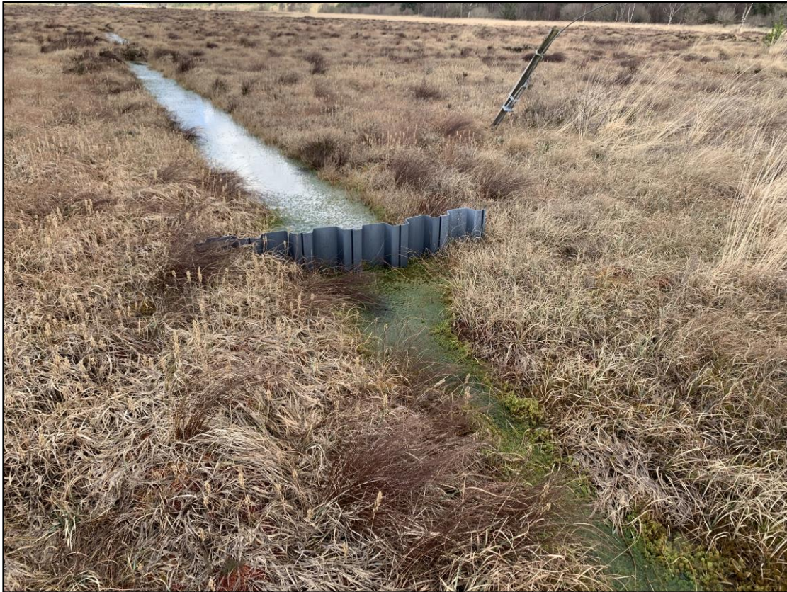
Figure 5.5 Example of plastic dam at Drumalough Bog
