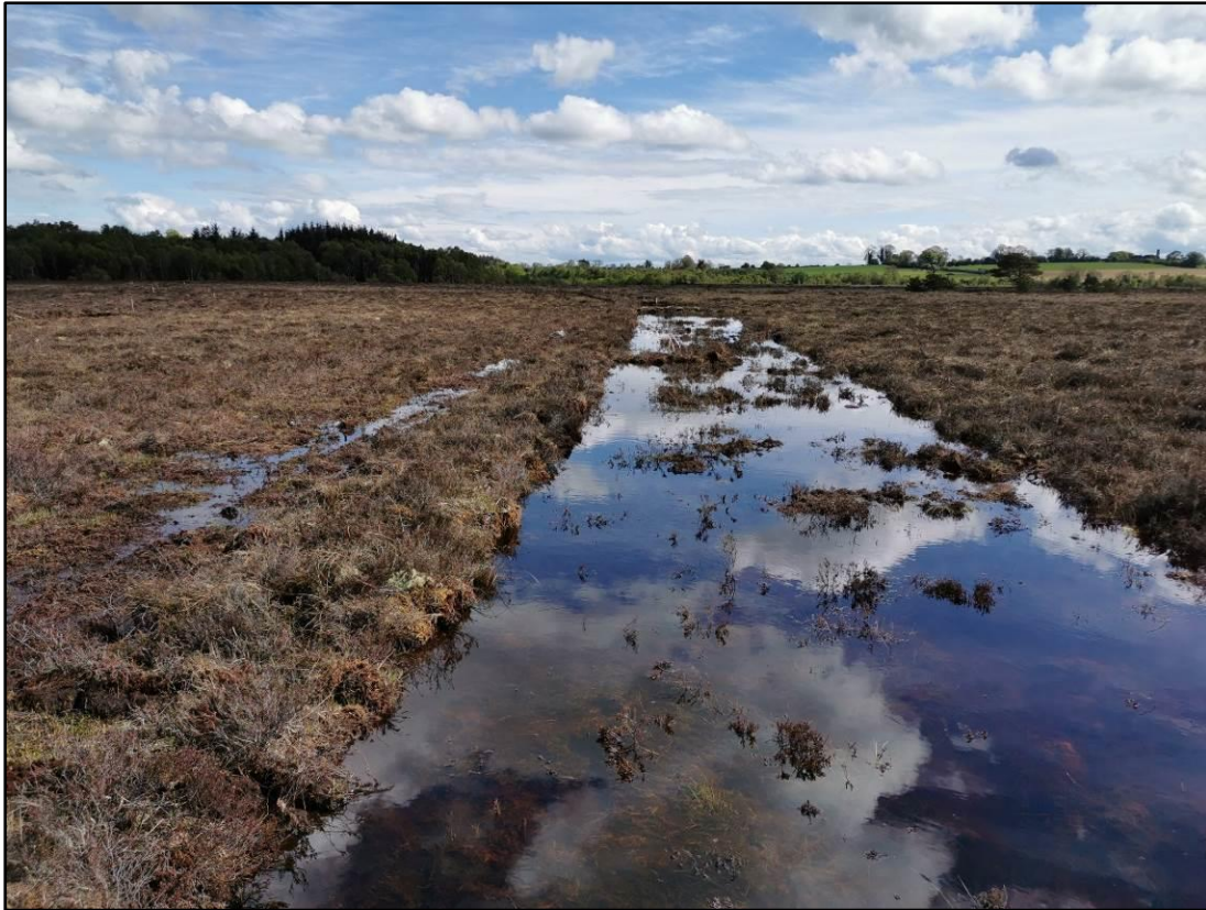
Figure 2.4 Example of contour bund constructed at Knockacoller Bog SAC, Co. Laois
