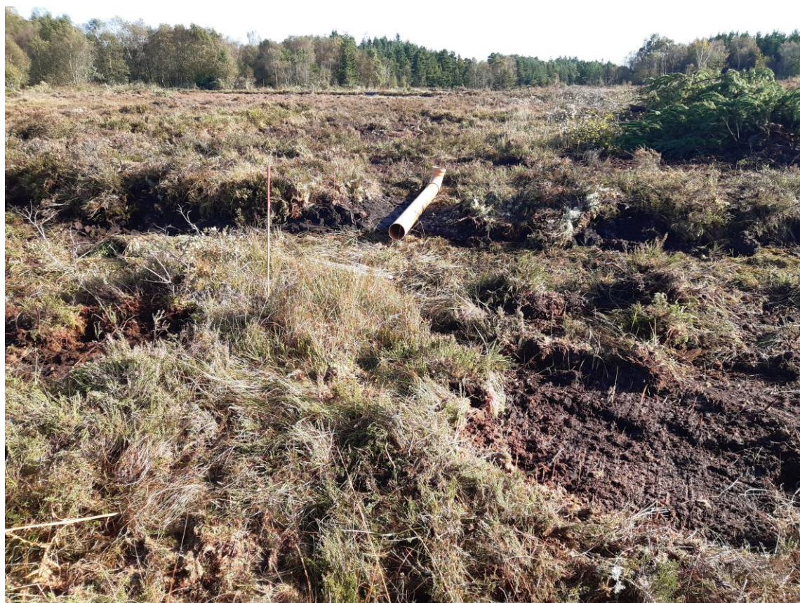
Figure 5.3 Example of setting out for piped weirs in a trench bund on the cutover. The bamboo is sprayed red
