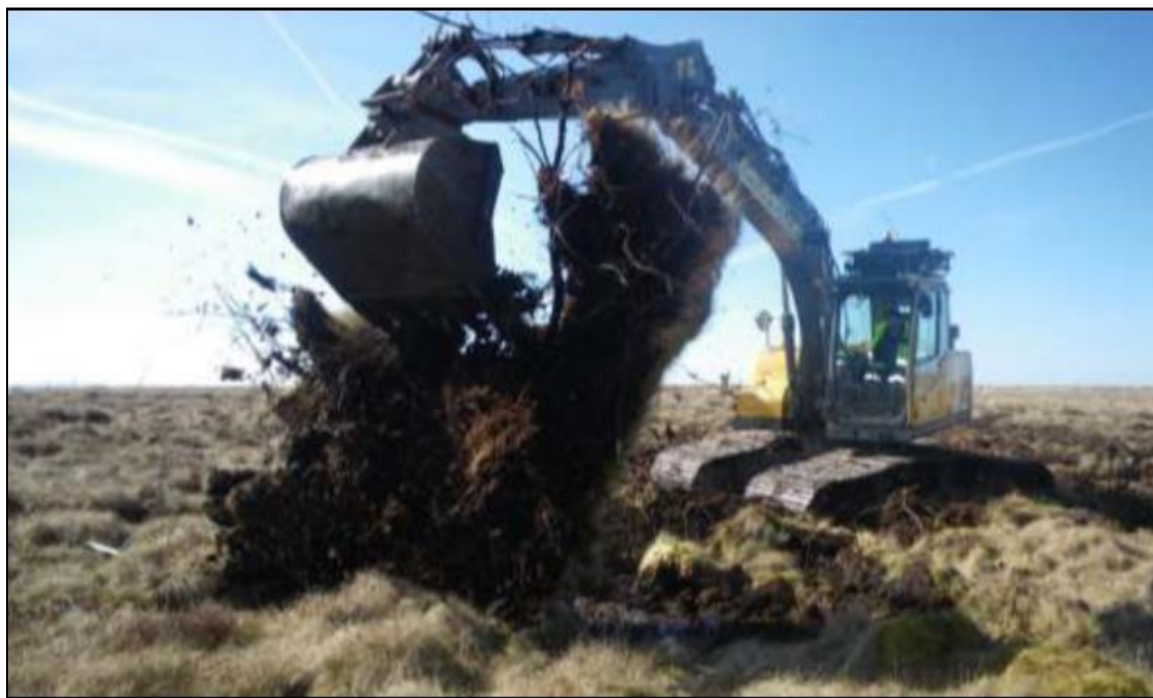
Figure 5.5 Example of stump flipping
