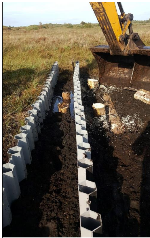
Figure 5.4 Example of large sandwich dam trialled on Carrownagappul
