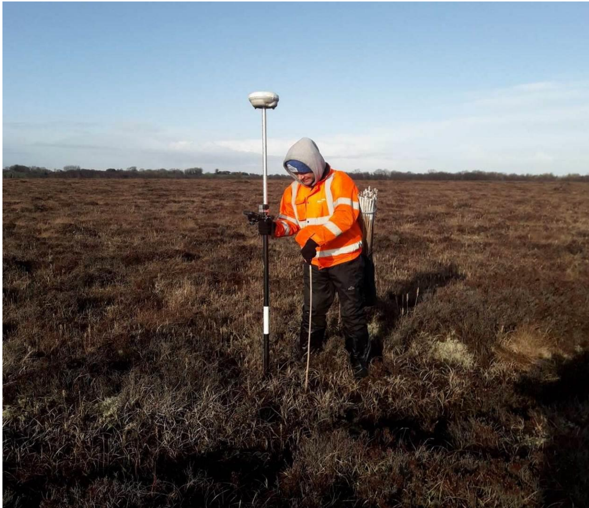
Figure 5.3 Example of setting out dams on an area of high bog
