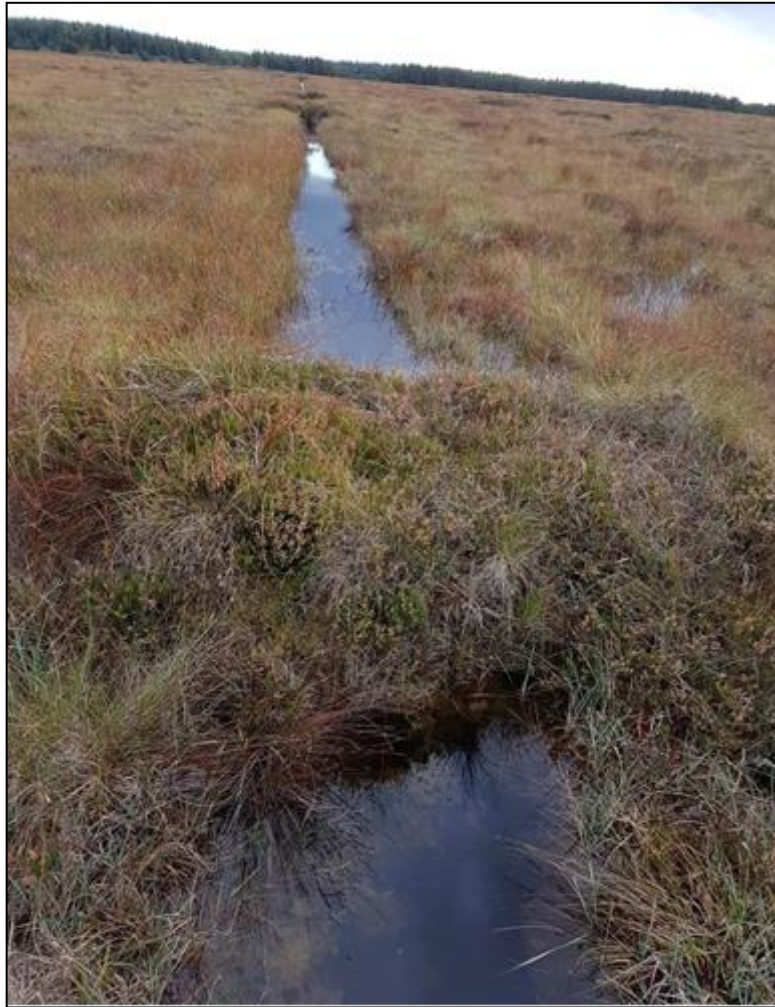
Figure 2.1 Example of a peat dam to block a typical high bog drain
