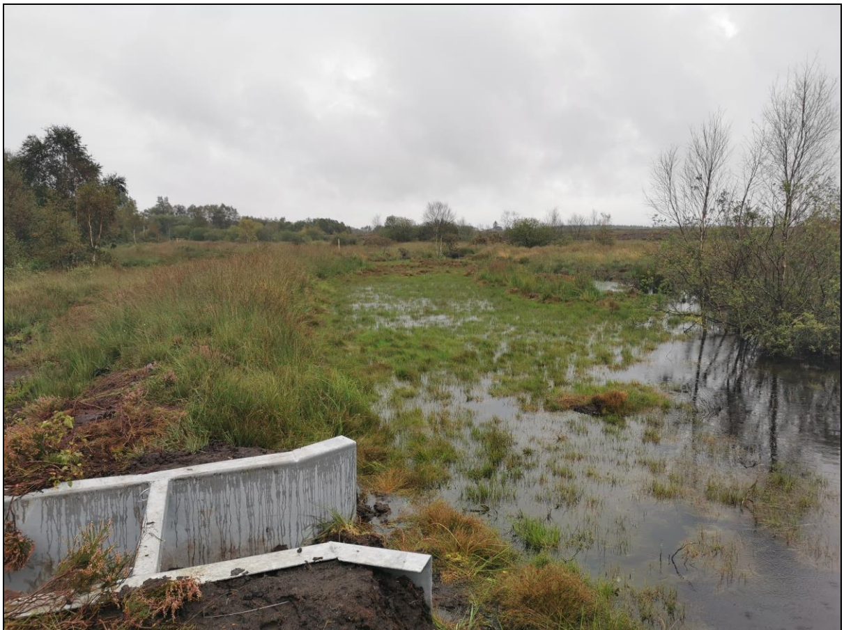
Figure 5.6 Example of bespoke outlet constructed for the large marginal bund/barrier dam on Ardagullion which has a set level to optimise rewetting of the cutover bog
