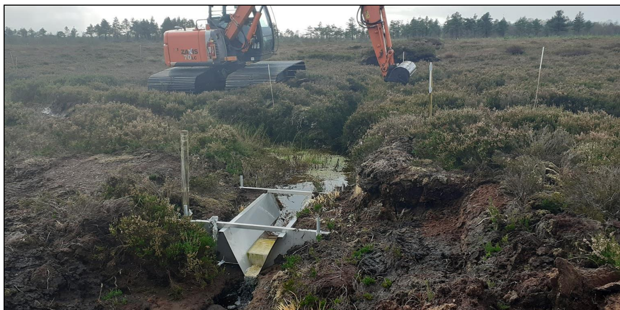
Figure 5.2 Example of bamboo sticks setting out dams on an area of high bog, with flume measuring flow rate of water off high bog in foreground
