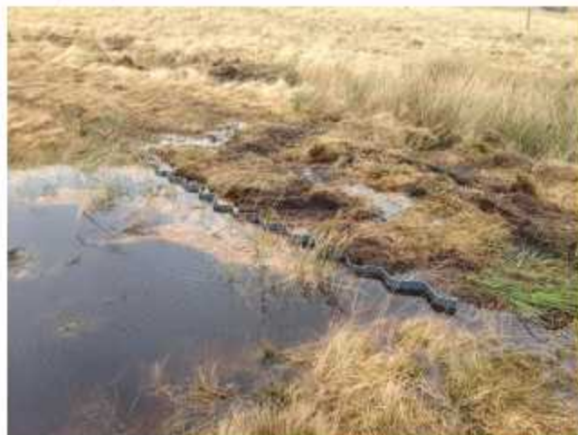
A plastic dam at another site. If sphagnum moss and other vegetation grows on the pool and dam it is a sign that you have built a healthy dam and ARB is developing well.
