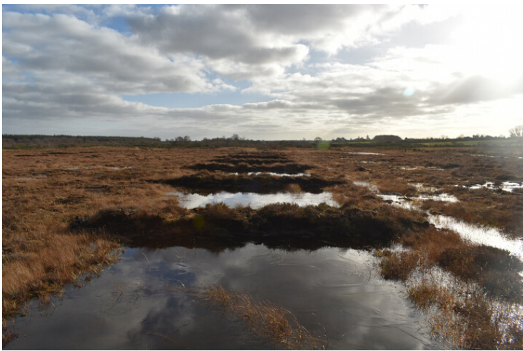
Well over a thousand peat dams have been installed on Carrownagappul Bog SAC, aka 'Galway's Living Bog' in Mountbellew. Here are some of the larger 2m dams that were required for some of the larger drains. They have stopped thousands of gallons of water being lost every hour from the site.
